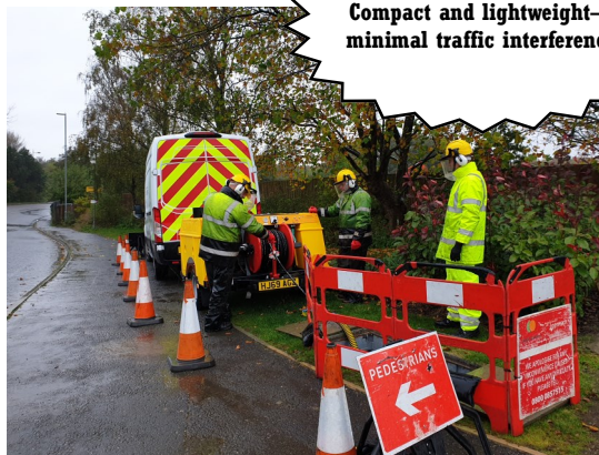
Setting up a Harben desilter on a main highway
