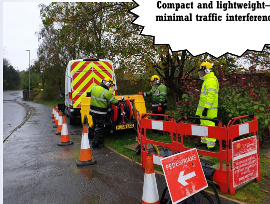
Setting up a Harben desilter on a main highway
