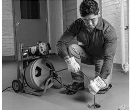
Figure 13 – In Operating Position, Manually Feeding Cable
