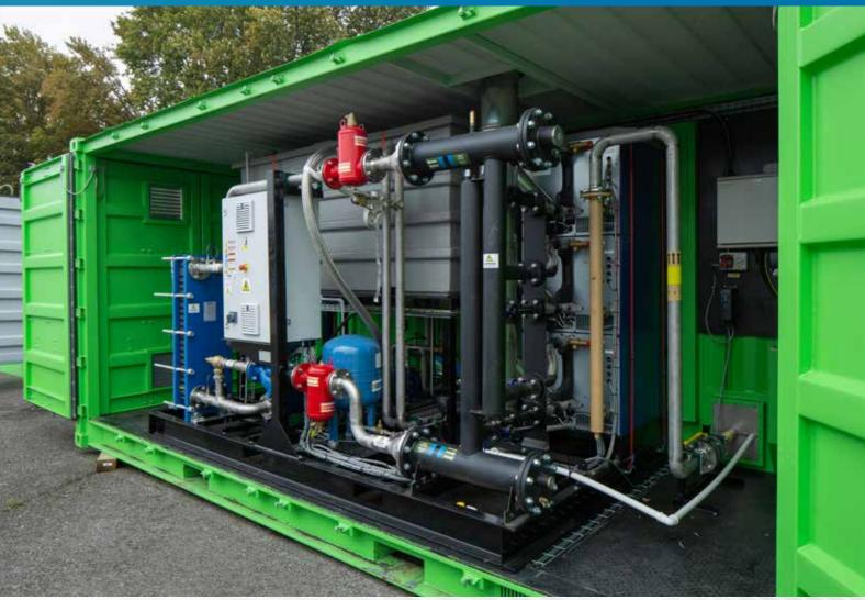
Serving for a more permanent installation, these modular designs allow for the customer to have very little down time whilst updating/renovating their plant rooms. Enabling the rooms to be permanent fixtures also allows the customer to utilise the old plant rooms for further building development.
